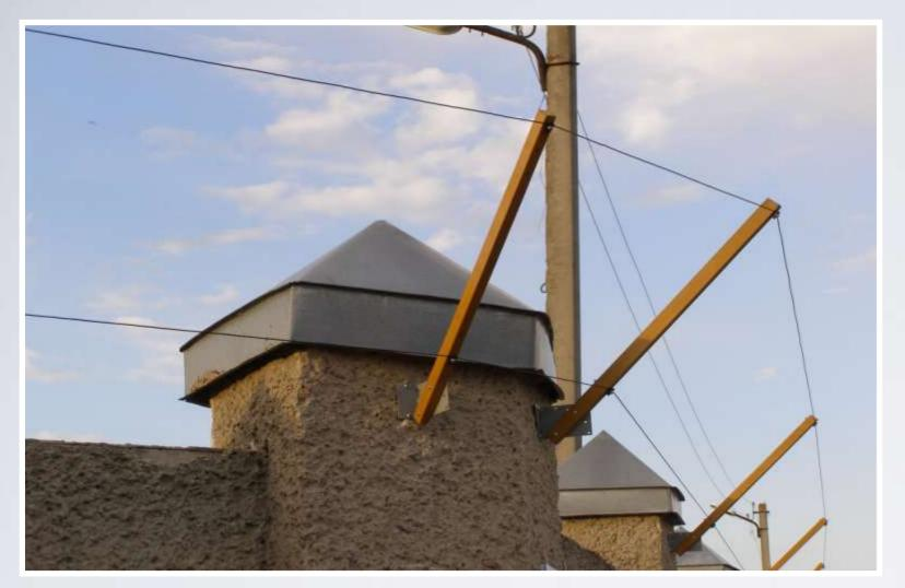
The detector permit Two separate types of installation, Visor and Ground. In the First option the detector is installed atop the boundary wall of the protected area, whereas the second option allows a detection zone to be created between the ground cable and the upper cable that is installed on fibre-glass poles.
